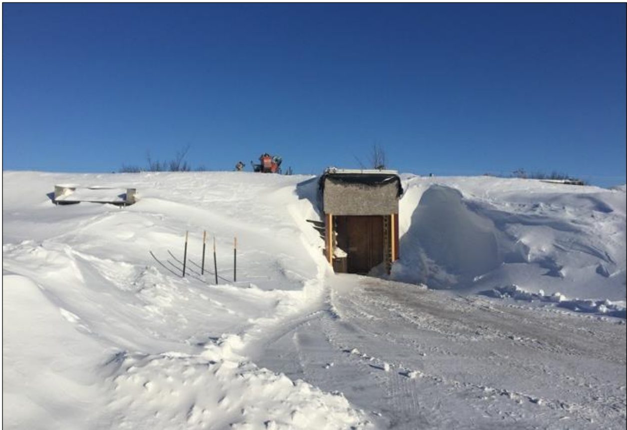
Figure 2. Produce Storage Bunker at Meyers Farm
